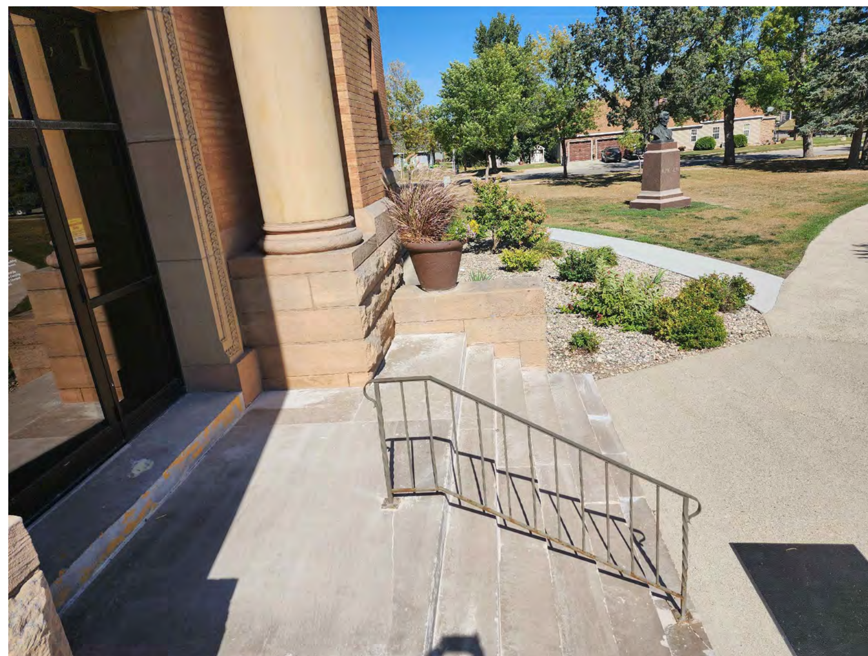
2 EXTERIOR STEPS - LOOKING NORTH A20 NO SCALE
