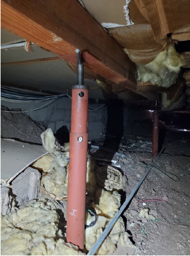
Photograph 7: Beam under floor trusses in Building 1.
