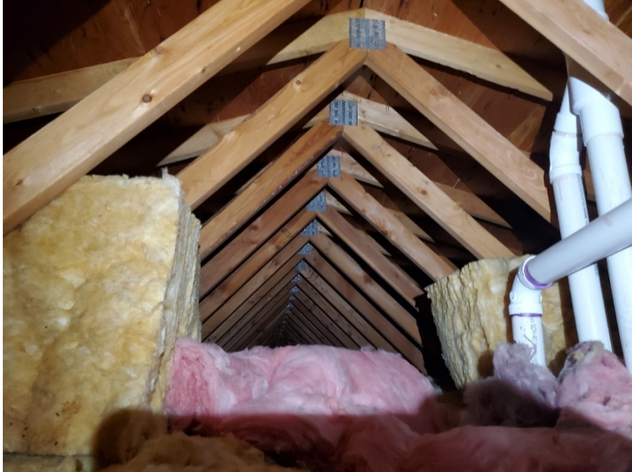
Photograph 5: Typical Roof truss applicable to Buildings 1-4.
