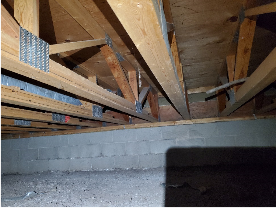
Photograph 3: Typical floor trusses from Buildings 1 and 2.
