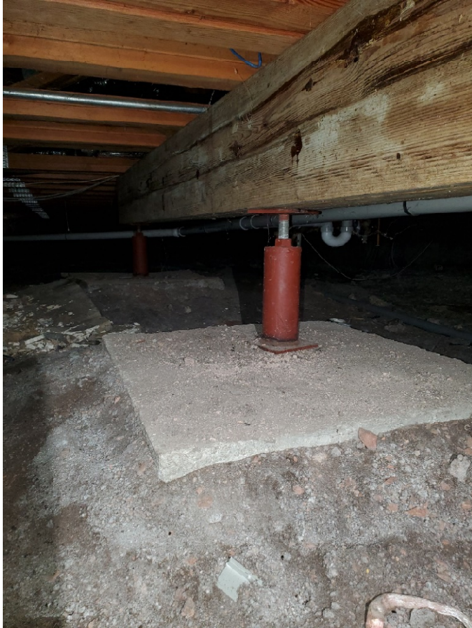
Photograph 8: Beam under floor trusses in Building 2.
