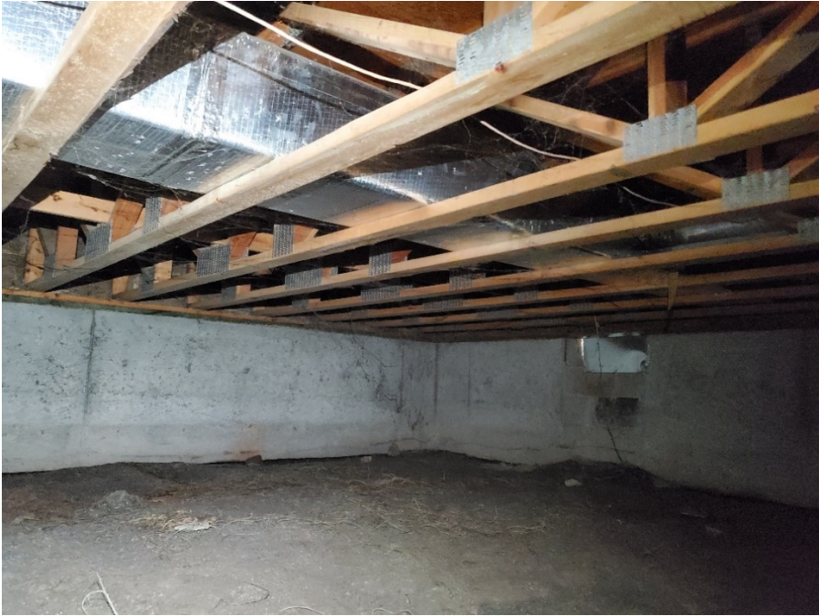
Photograph 4: Typical floor trusses from buildings 3 and 4.
